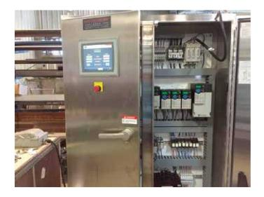
and the sludge—the sludge then forms into small popcorn size balls in the water. The variable speed mixer allows operators to easily change the mixing energy which helps ensure the best possible flocculation.
