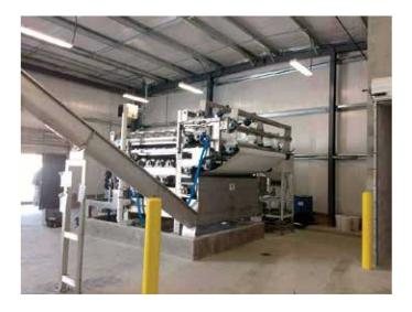
Sludge cake monitoring system: A unique OR-TEC add-on feature which constantly monitors and detects the sludge being discharged from the Belt Press. If no sludge is detected for one minute, this entire system shuts down and an alarm is activated.
